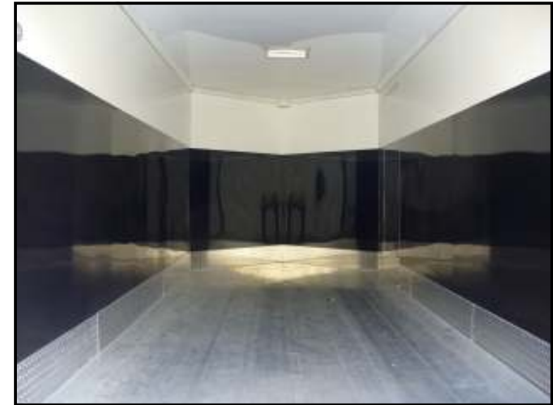
Aluminum lining on walls and ceiling
